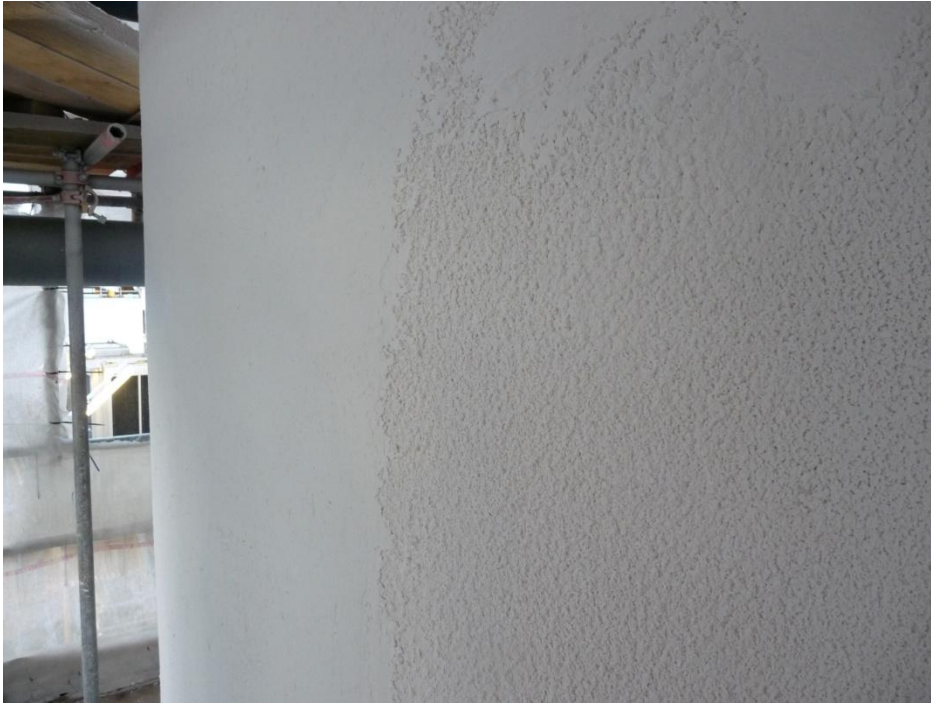
Surface partly troweled (left)
