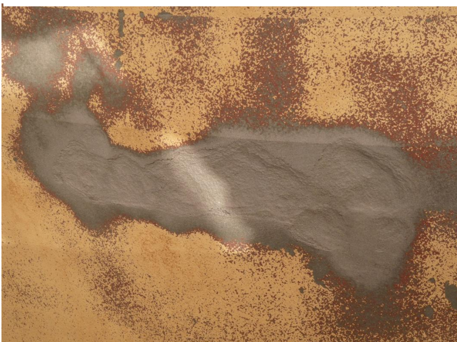
Blasting until bare metal on heavily corroded areas
