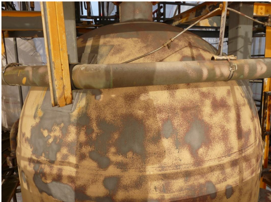
Sweep blasted surface before application
