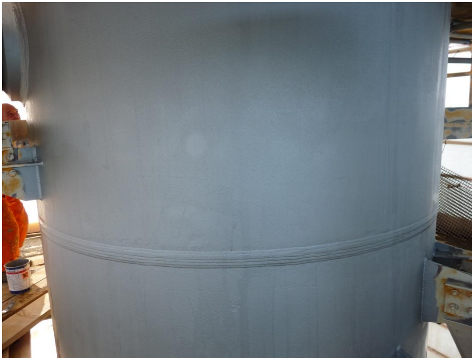
Second section from top completed
