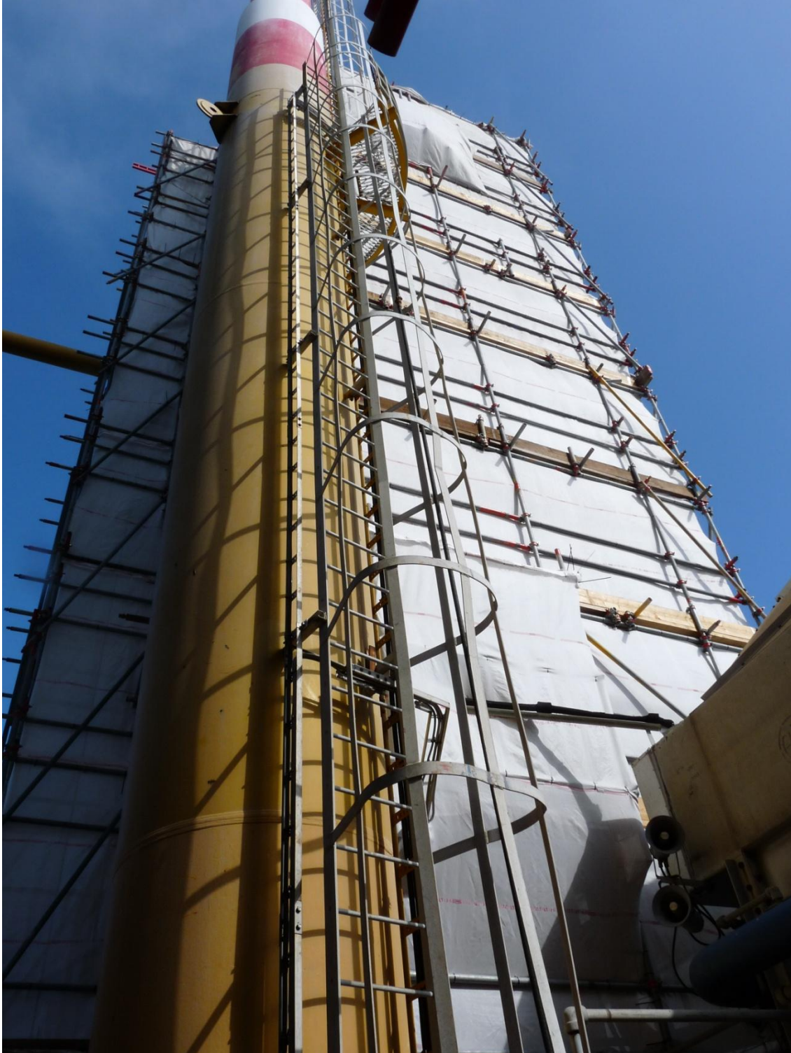
Vessel covered with scaffolding and tent
