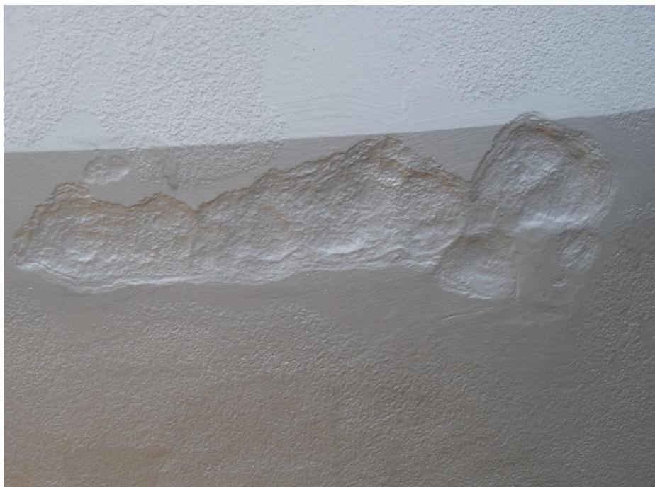
Rust Grip applied on heavily affected areas
