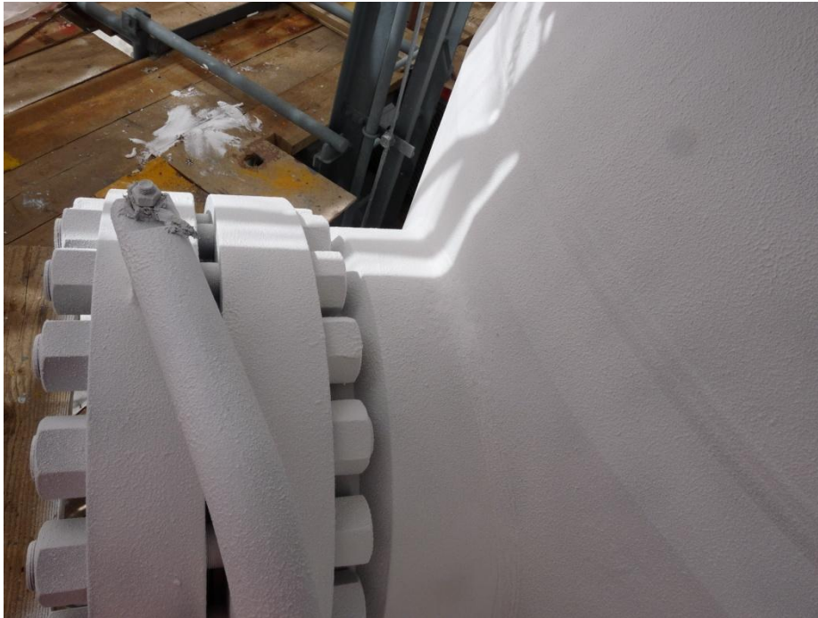
HSC applied on manhole
