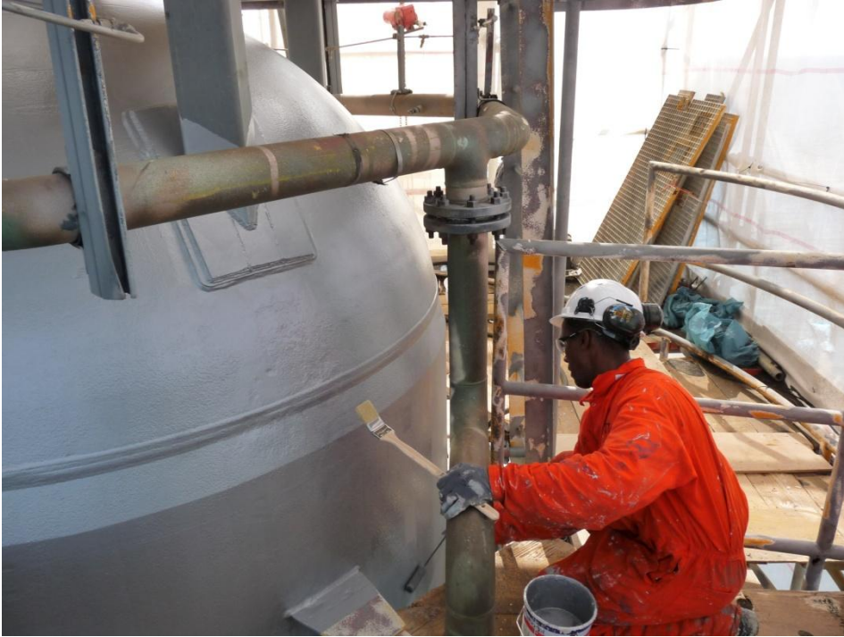
Application of Rust Grip by roller and brush
