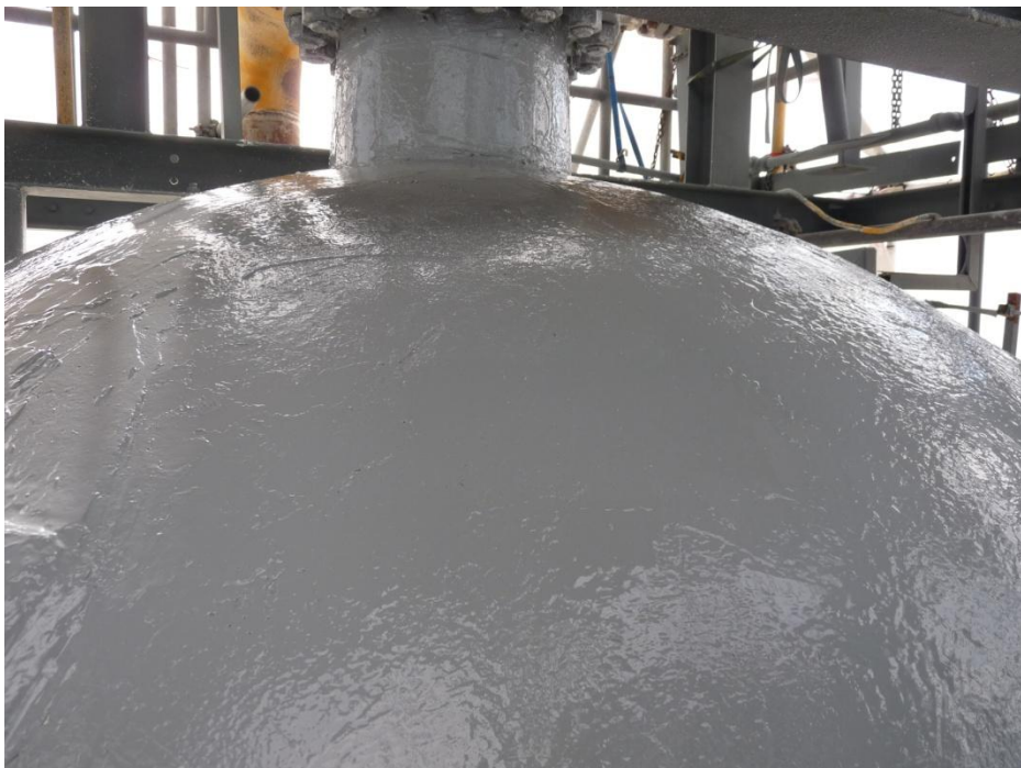
Top completed with Enduroof
