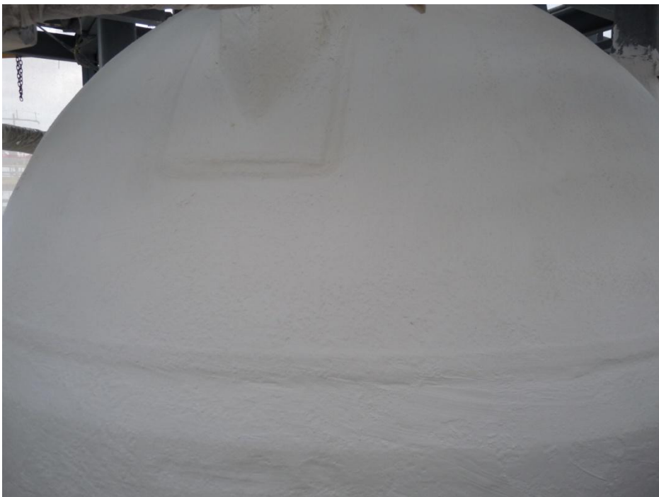
Top level after trowelling
